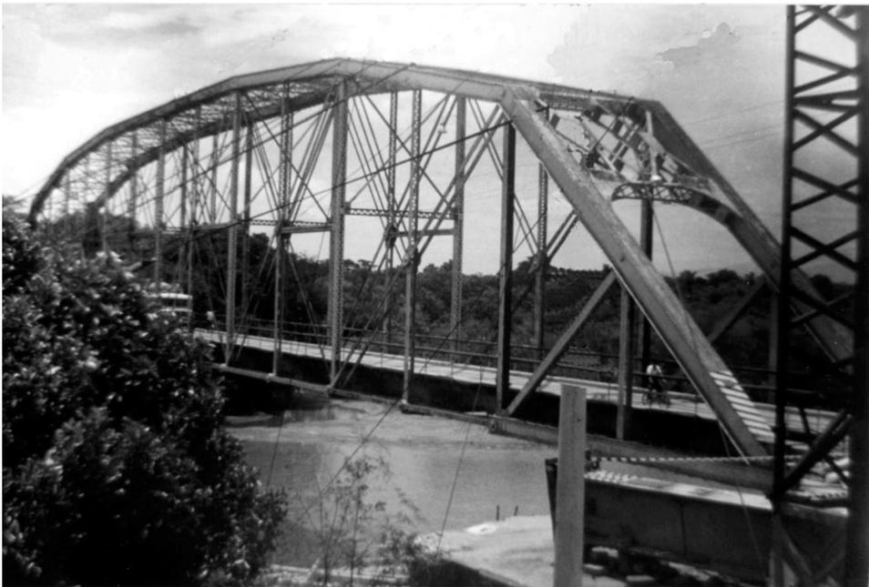
Saldaña (Through, pin-connected) (FC Tolima Huila-Caquetá o Girardot)
