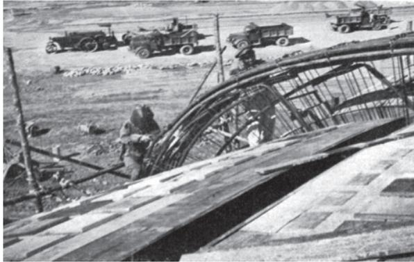
Figura 5. Imagen del armado del punto de intersección entre el brazo superior e inferior publicada en *Architectural Record*, 1:104. July (88-93). El pie de foto manifestaba que: Here may be seen the powerful reinforcing bars wich take the tensional stress of C-curved vertical frames. Note also the preparation for coffering the thin canopy membrane ...
